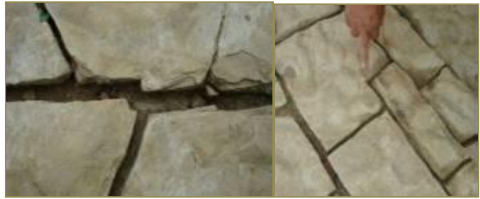
AT SB1 DETAILS SHOWING THAT THE TILES WERE CAREFULLY SET TO FIT.
